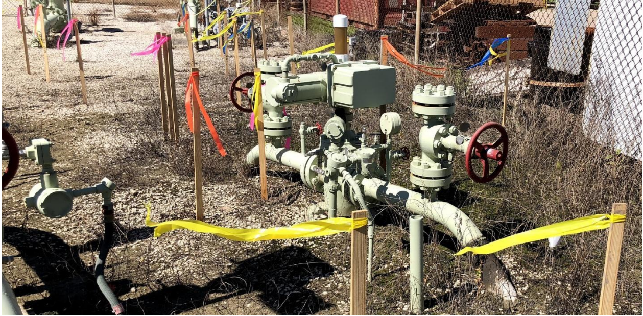
Figure 7 One Call Stakes at Valve Site
